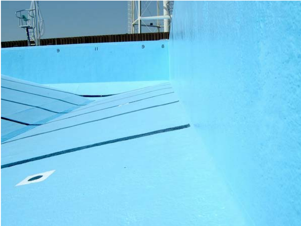
Photo 4: Permafex Project – After Installation of Elastomeric Liquid Rubber Coating
