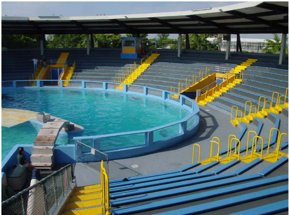
Photo 8: Versaflex Project – Finished Installation of Polyurea Coating at Killer Whales Tank
