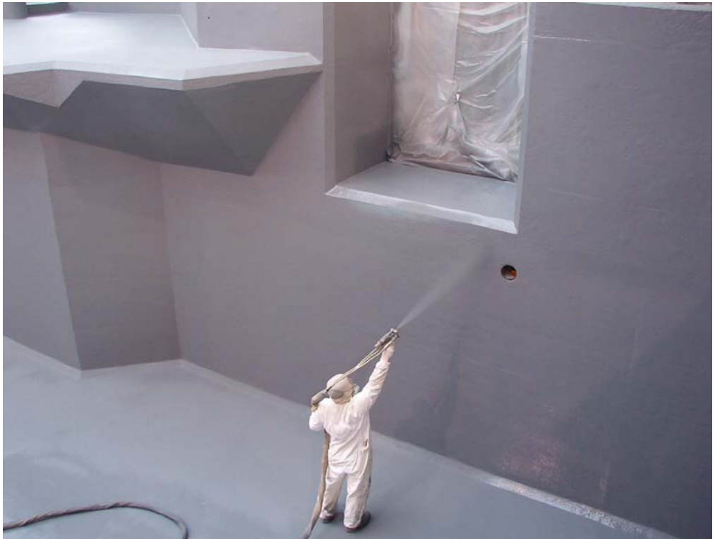
Photo 5: Versaflex Project –Installation of Polyurea Coating at Dolphin Tank
