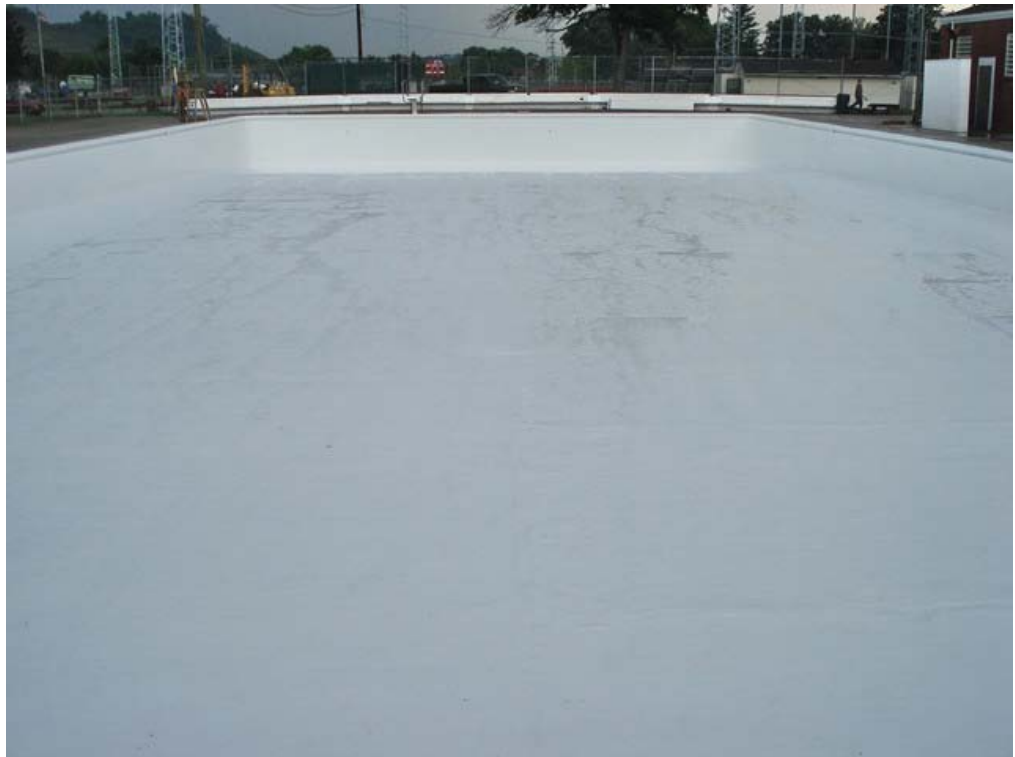
Photo 2: Permafex Project – After Installation of Elastomeric Liquid Rubber Coating.
