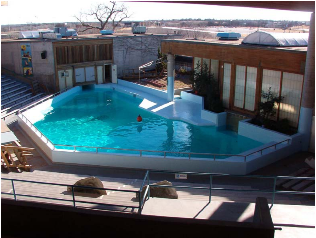
Photo 6: Versaflex Project –Finished Installation of Polyurea Coating at Dolphin Tank
