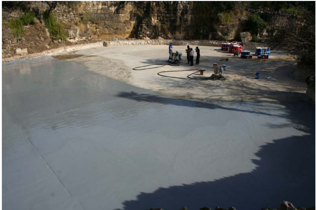
Photo 7: Versaflex Project –Installation of Polyurea Coating at Water Feature
