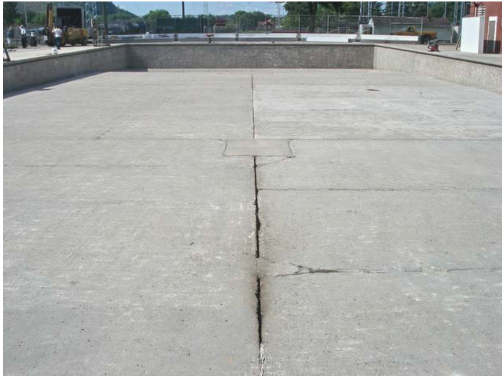
Photo 1: Permafex Project – Before Repair and Application of Elastomeric Liquid Rubber.
